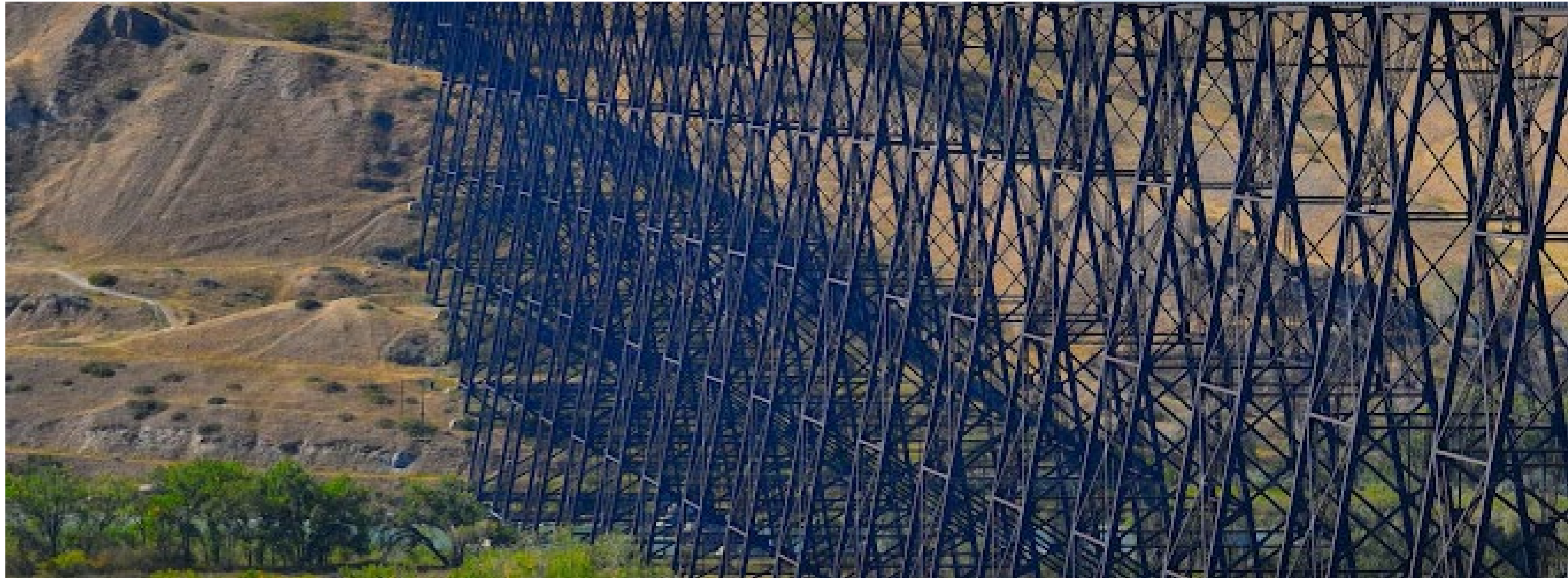
High Level Bridge / Lethbridge Viaduct
